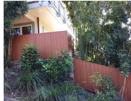
Fence installation on uneven grade
