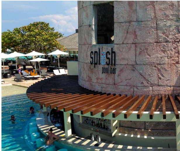
The battens used to create the roof for this pool bar not only provide shelter for the staff and patrons, but they also offer a truly tropical feel.
